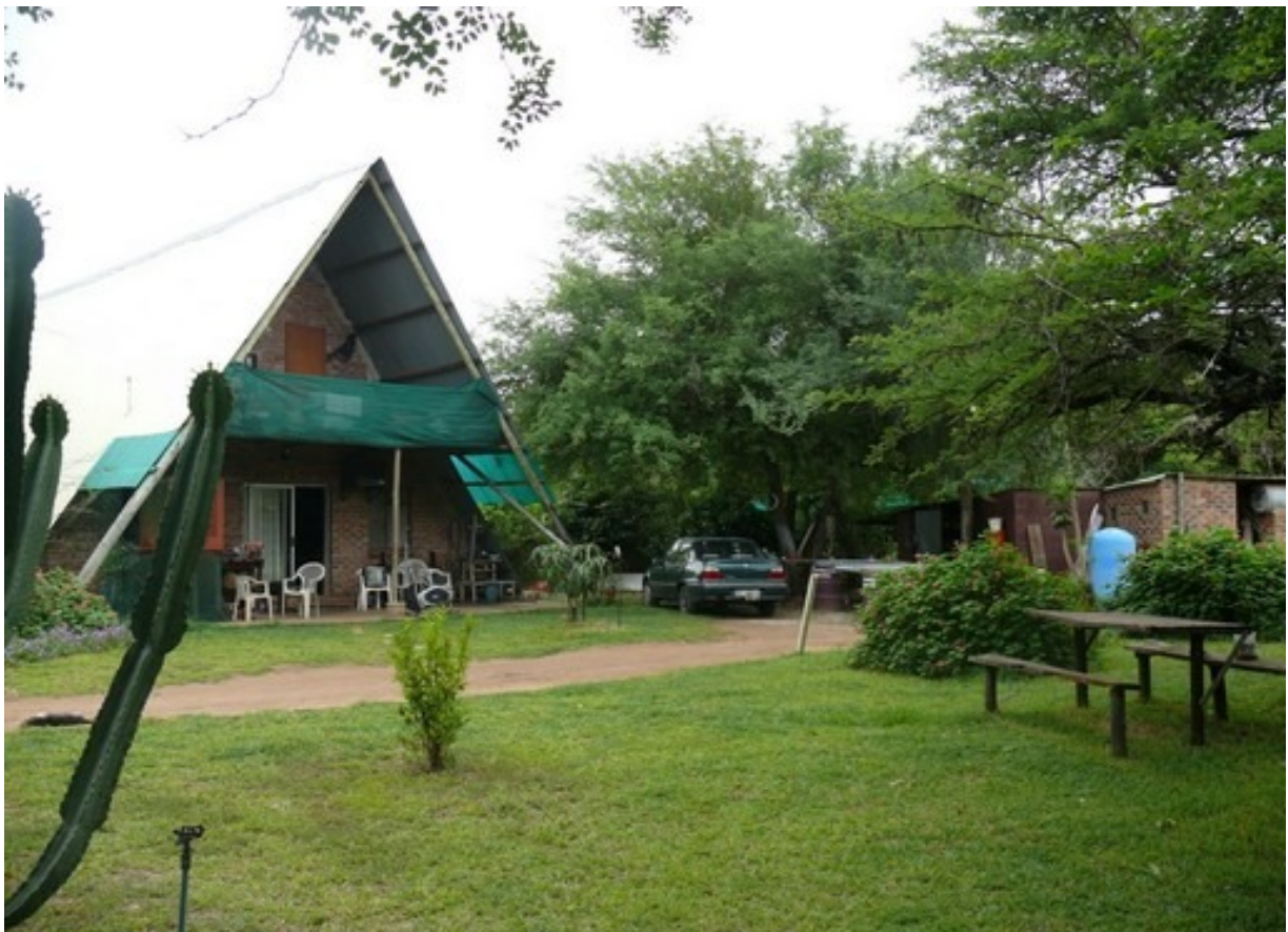
This is the main A-frame house. The workshop and storage areas are to the right.
